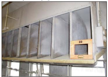
The # 23 stained and polyurethane coated paper box door is shown in place. It now has a label holder with pull. Other paper boxes and the rows of first class letter slots are shown in photos. Below, a handsome, portable sorting tray that was made, stained and polyurethane coated at home.
