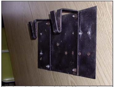
This shows the brackets on the back of the number for hanging it below the signal tower.
