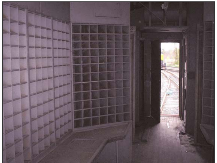
View of one end of the interior of the car, showing one of the two sides lined with pigeon holes.
