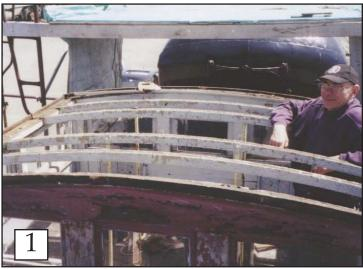
Franz Gerencir)then proceeded to take the entire cupola apart. As suspected, there was extensive wood rot. All of the pieces needed replacing except the roof trusses. These were rebuilt (see photo 2, before and
