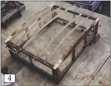
on a concrete platform (see photo 4). This gave us a good idea of how to complete the reconstruction of the cupola with new wood.
